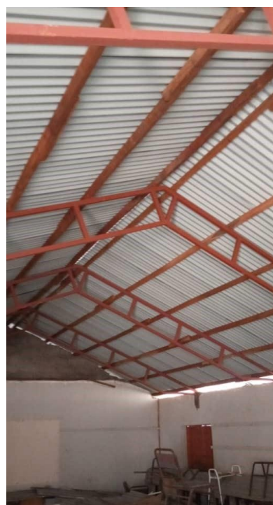
New Roof St. Peter's S.C. 2021.
