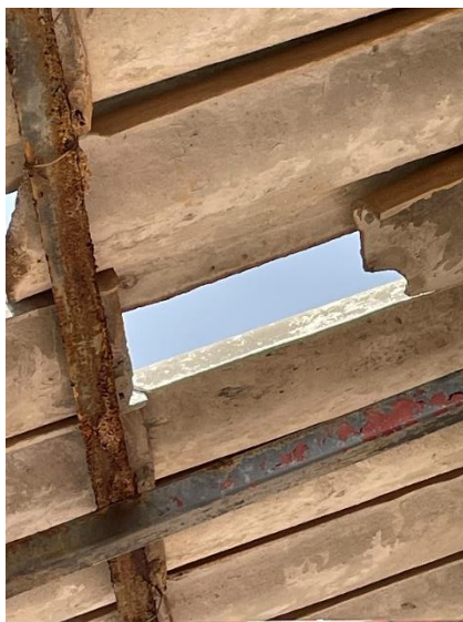
Baked Clay tiles crumbling. New Roof required in St. Francis' Nursery school.
