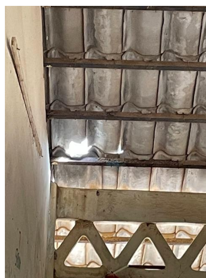
Baked Clay tiles crumbling. New Roof required in St. Francis' Nursery school.
